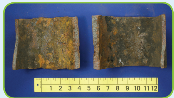
Cross section of extracted pipe sample from site #7
