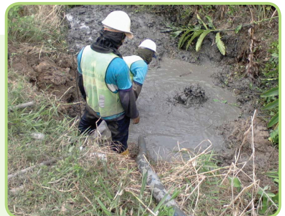
JCSB crews expose the leak that was non-invasively located by Echologics.
